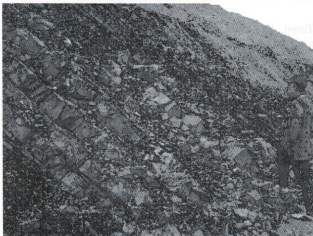
Fig. 10: Highly jointed sandstone and mudstone beds oriented parallel to slope face at Km 38
