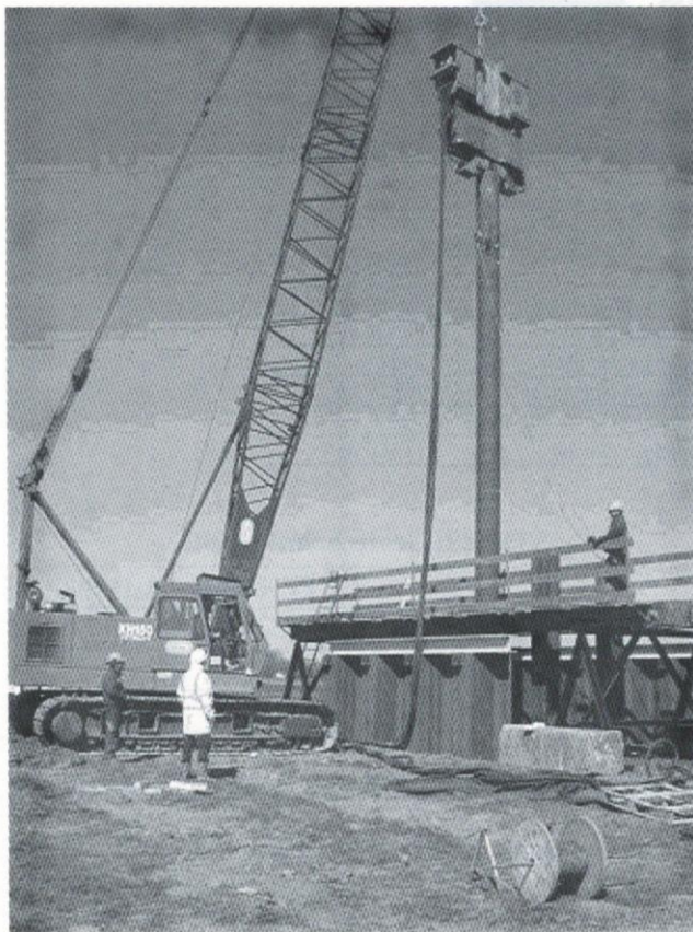
Fig. 6: Driving the pile
