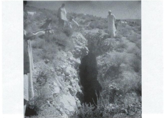
Fig. 6a: A deep and wide fissure in the Kirthar Formation
