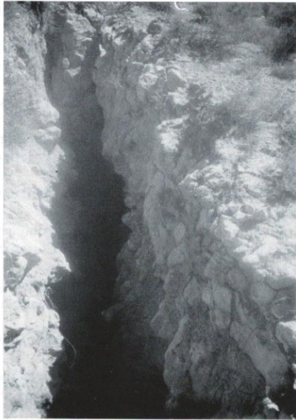
Fig. 6b: A wide fissure in the Kirthar Formation
