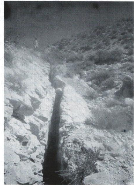
Fig. 6c: An extensive fissure in the Kirthar Formation
