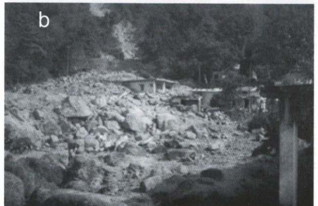
Fig. 7: Jyotinagar Landslide in Butwal, a: landslide scars, b: damaged structures
