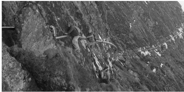
Fig. 3: Construction of the water pipe from Gyajo Khola, Namche Bazar area.
