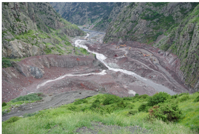
Fig. 13: The Terek River with the Daryal hydro-electric power station under construction in the distant view on June 10, 2014. Breaching of the debris rock-ice flow deposits of the Kabahi River.
