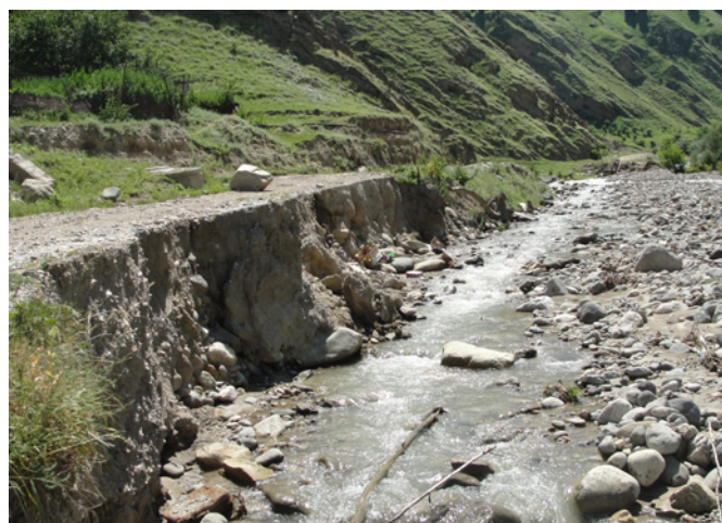
Fig. 10: Lateral erosion of the right bank of the Gestanty River as a result of a water rock flow on May, 21, 2014; a road to the potable water intake for the settlement of Bylym was destroyed.
