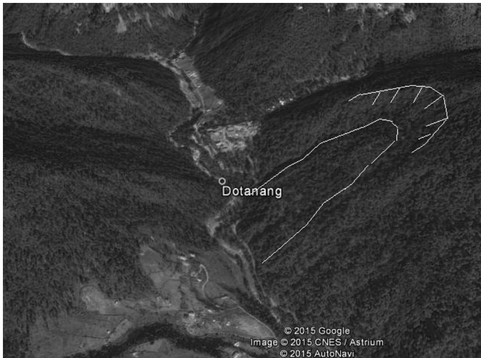
Fig. 13: Bird view of potential landslide ‘No. a’ (depicted from Google Earth).
