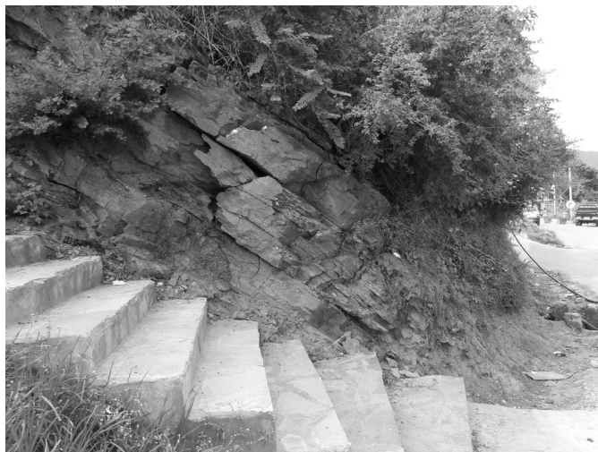
Fig. 19: The side view of ‘No. b’ which shows cuesta and has regular discontinuities.
