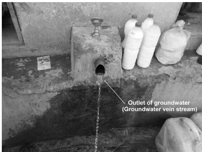
Fig. 18: The fountain of groundwater vein stream served as drinking water in ‘No. e’.
