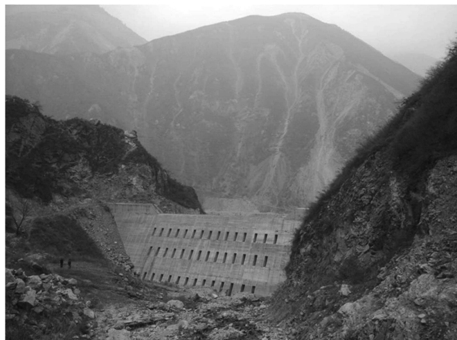
Fig. 7: The new-built silt arrester at the exit of the Mozi gully
