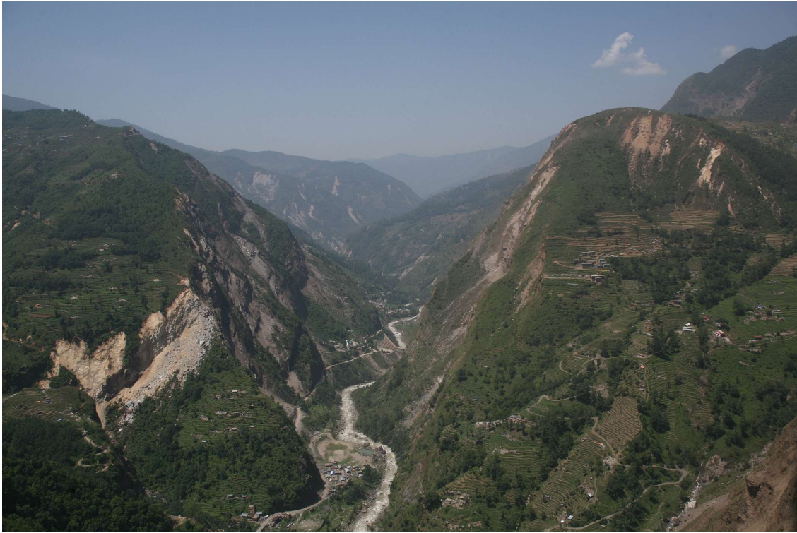
Fig. 6: Shallow landslide triggered by the Nepal Gorkha Earthquake 2015 along the Bhote Kosi Gorge
