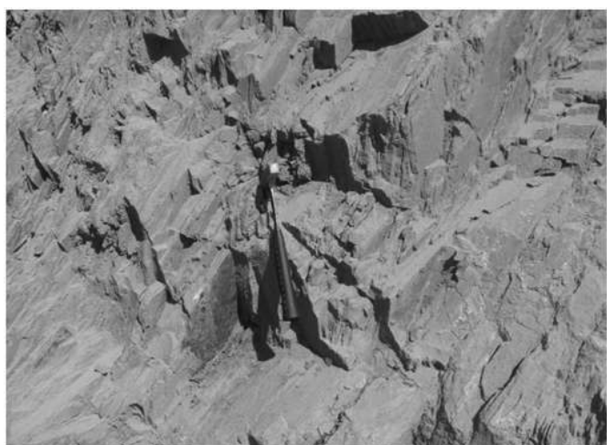
Fig. 6: Photographs of thinly-foliated and jointed black slate of the Tupkan Slate observed at the Tupkan village
