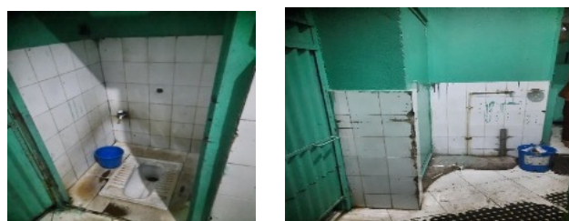
Picture 3: Public Toilet of Ratnapark
