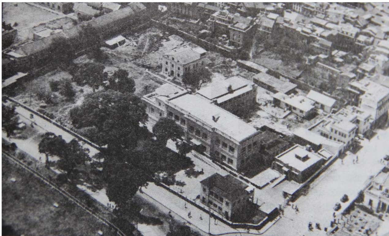
Figure 2: Aerial picture of the Bir Hospital compound showing its different components 8
