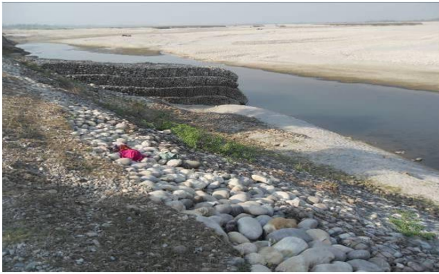
Figure 13: Spur protection embankment (Mahakali River)
