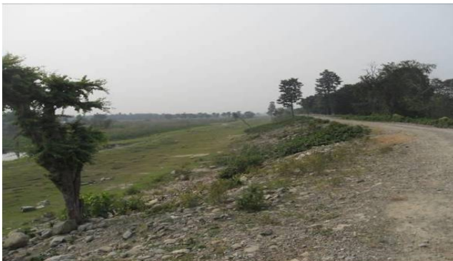
Figure 9: East embankment (Koshi River)
