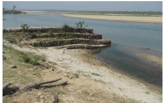
Figure 11: Isolated spur with no revetment (West Rapti River)
