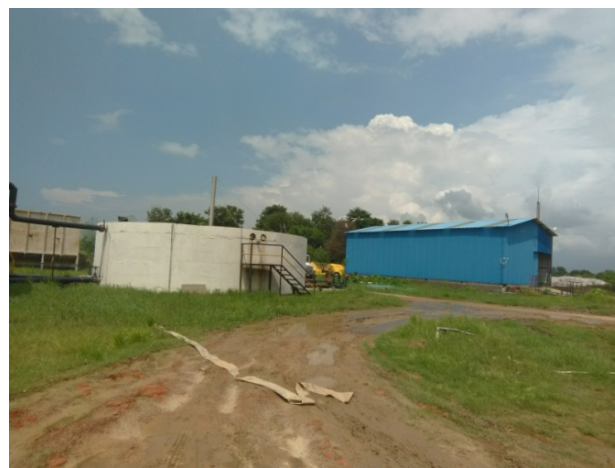
Figure 4: Biogas plant in Ramgram Municipality
