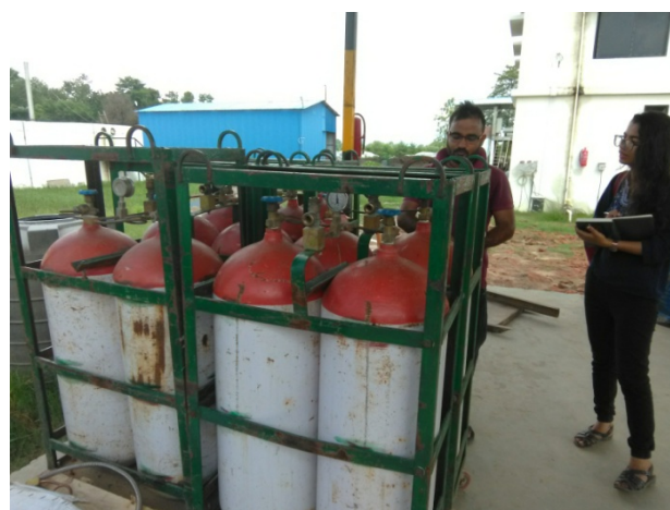
Figure 6: Biogas filled in containers
