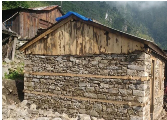
Fig. 7: Newly constructed house in Haku with timber gables and timber bandings
