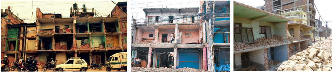
Fig. 1: Dismantled buildings during Road Widening Project in Kathmandu.
