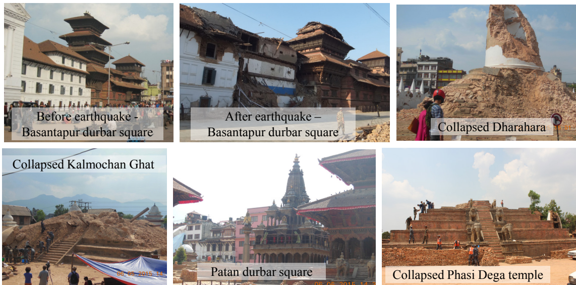
Fig. 7: Typical failure observed in heritage structures in Kathmandu Valley.
