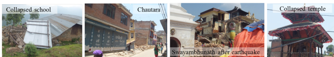
Fig. 15: Damage observed at the top of hill or along the ridge
