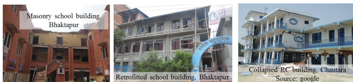
Fig. 8: Performance of the school building during the earthquake
