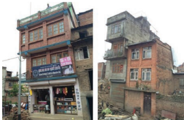
Fig. 11: Vertical irregularity in Sankhu buildings
