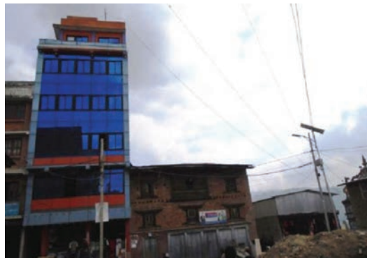
Fig. 12: Neighboring buildings of different heights in Sankhu
