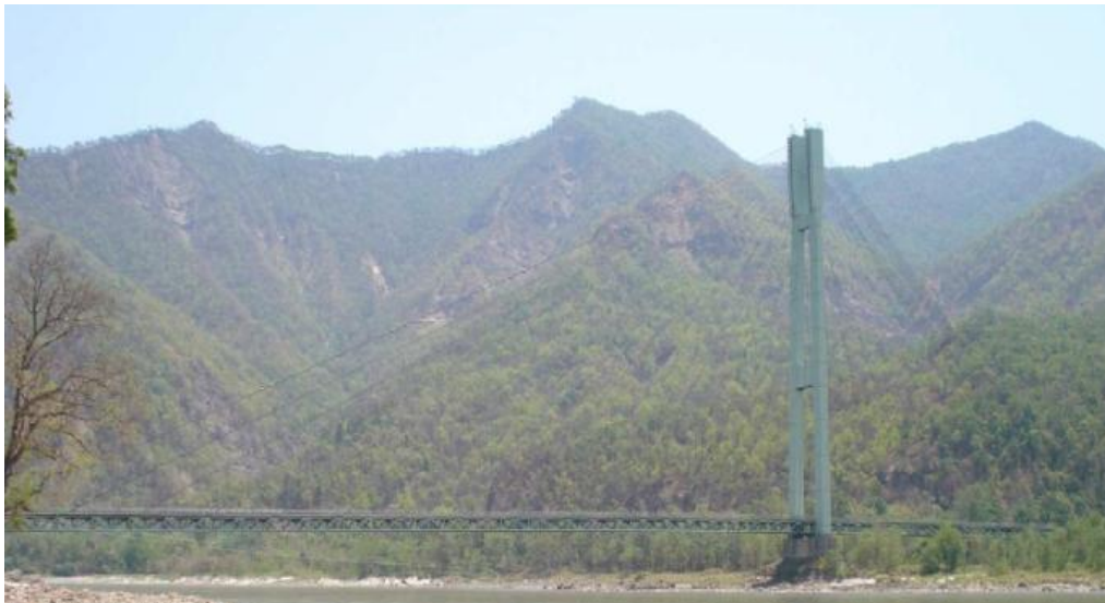
Figure1: Image of Karnali Cable-stayed Bridge stayed
