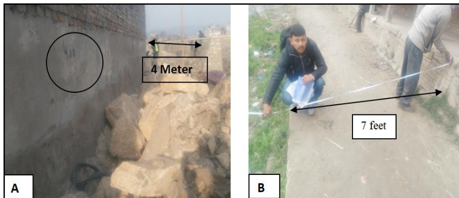
Figure 8: Encroachment by the Garment and Washing Factory (A), Pati build at the Bank of river at Barahisthan (B)
