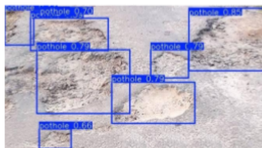
Figure 11: Pothole Detections on Sri Lankan Roads 3
