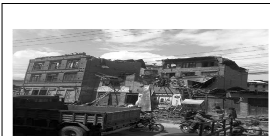
Fig. 29: Roof failure of building.
