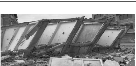
Fig. 30: Overturning of a 7 storey tall building in Kapan area, Kathmandu.
