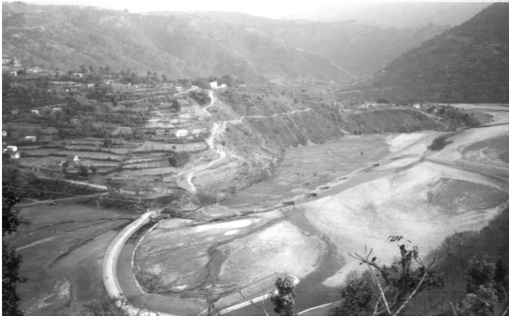
Fig 2 Downstream end showing photograph of 12MW Jhimruk Hydropower Project (Source: Butwal Power Company (BPC))
