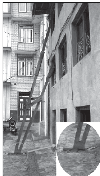
Figure 15: Protecting building with small wooden support
