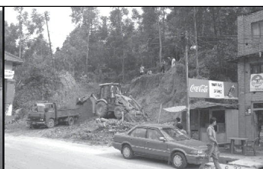
Figure 17: The toe cutting of the slope for construction
