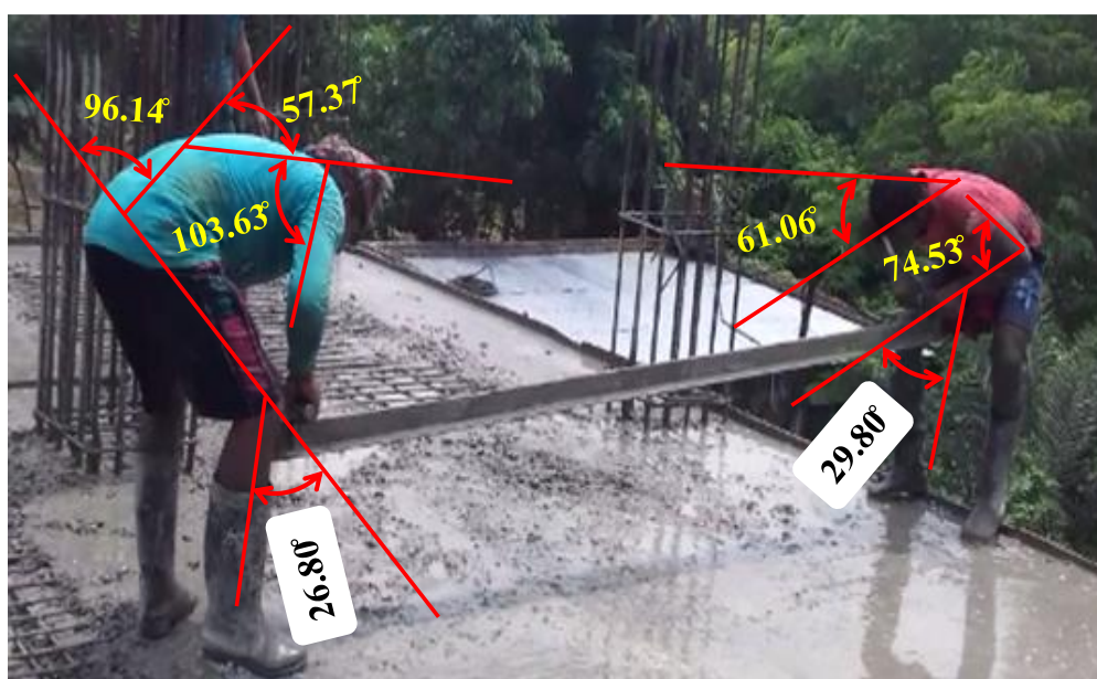
Figure 13: Body posture of the concrete-layer
