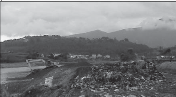
Plate 5. Bagmati River, ditch making at the bank and pile of waste ready to bury
