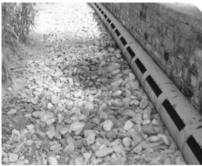
Figure 5(b). Slotted Pipe Inlet (UN-HABITAT 2008)
