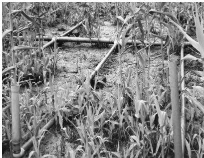
Figure 5(d). Network of Perforated Inlet Manifolds in VFB (Kathmandu University, Nepal).
