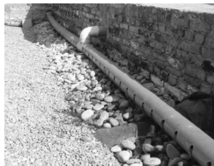
Figure 5(a). Perforated Pipe Inlet (UN-HABITAT 2008).
