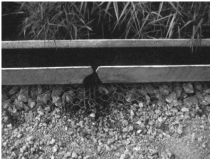
Figure 5(c). Close View of Channel inlet (Cooper et al 1996, cited in UN-HABITAT 2008) .
