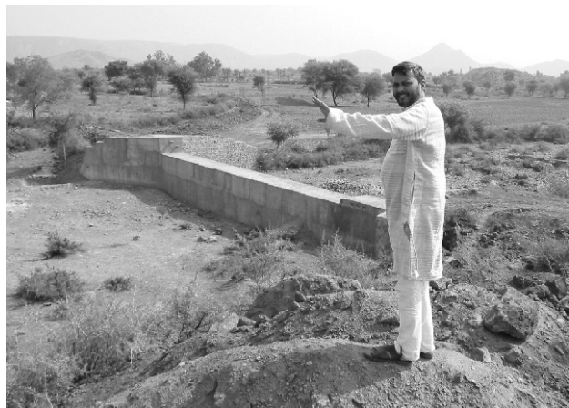
Mr. Rajendra Singh showing a water harvesting structure
