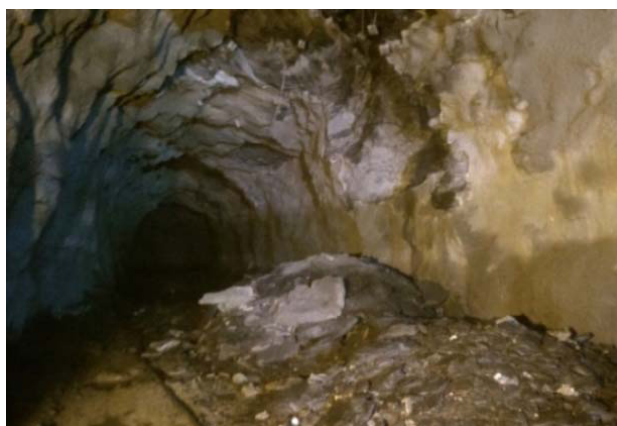
Figure 12. Post excavation dilation resulting in slabbing
