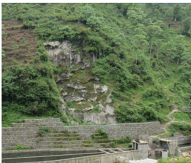
Photo 4: Stabilization of slide
