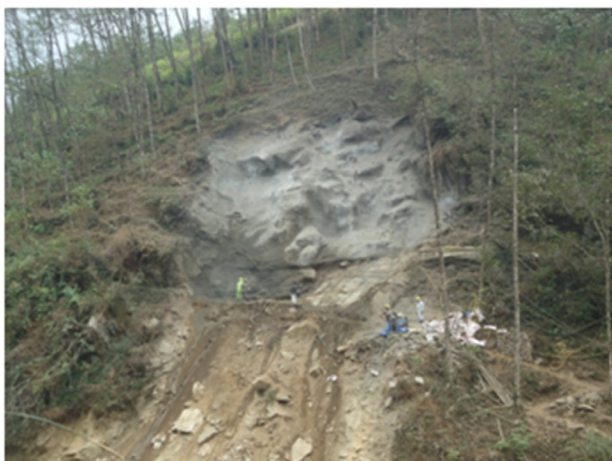
Photo 3: Application of shotcrete on slope
