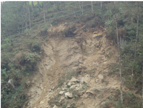
Photo 2: Removing loose material from top of landslide
