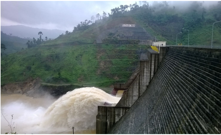
Figure 2: Roller compacted concrete (RCC) main dam at ST2 HPP.
