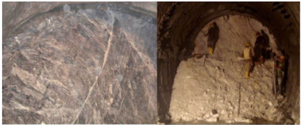
Figure 3. Rock mass condition at different chainage along the headrace tunnel
