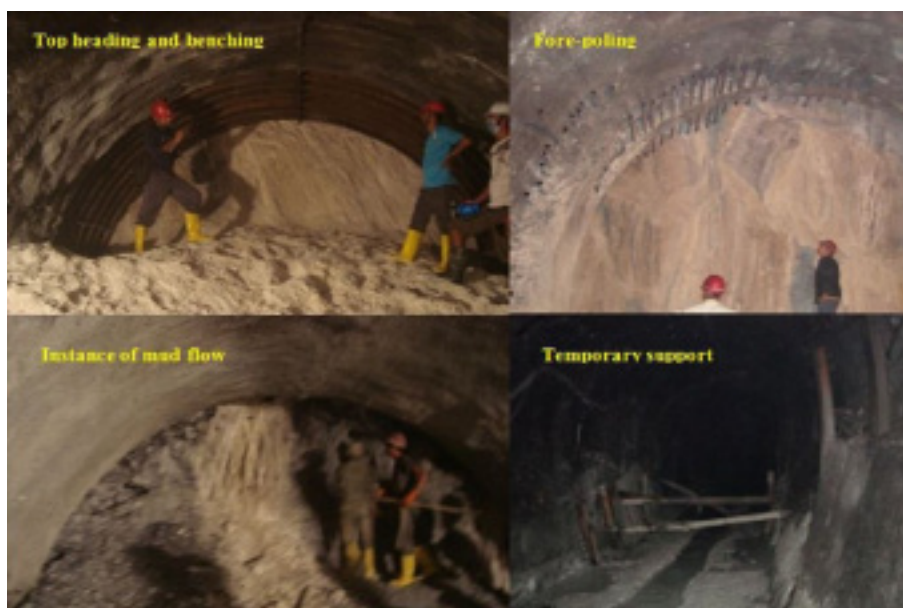
Figure 5. Several instances of tunnel excavation in CHEP at squeezing part
