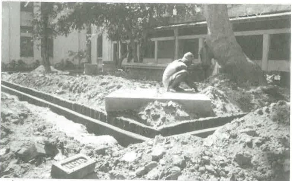
Rain Water structure in under construction at Santiniketan Central Library, Visva-Bharati
