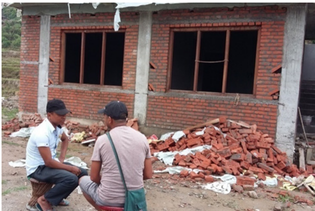
Figure 4: Informants Constructing Earthquake Resistant House
