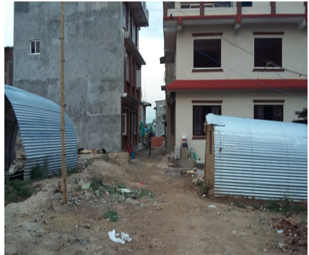
Figure 8: Housing Structure after Earthquake in the Same Place
