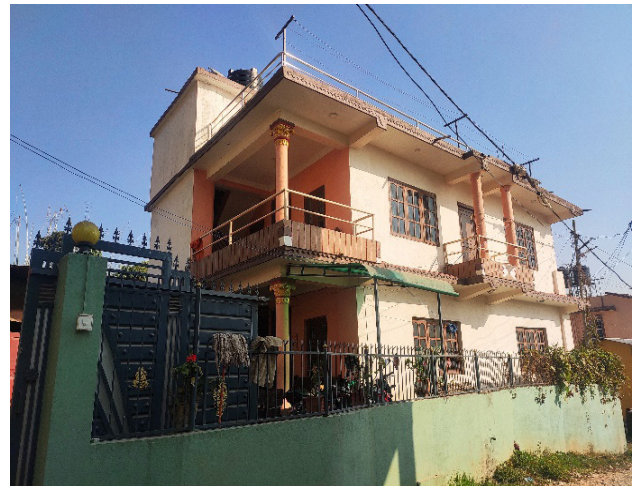
Figure 6: Affected Structure after Retrofit
