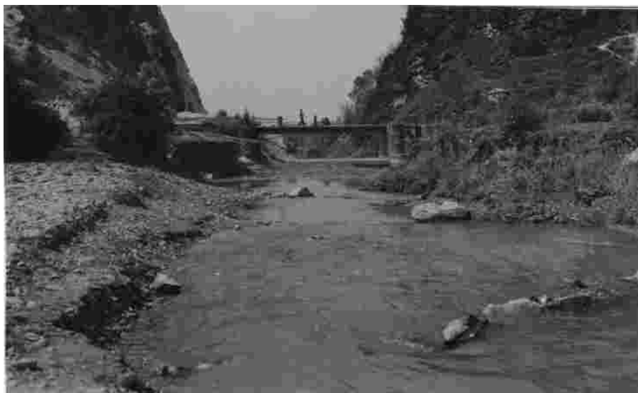
Fig. 8 Photograph showing suggested dam and reservoir site in the Kodku Khola
