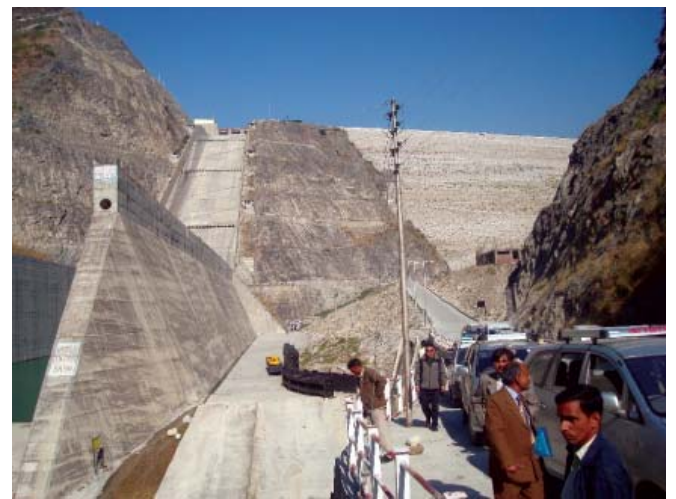
Photo 3. Downstream View of Tehri Dam
